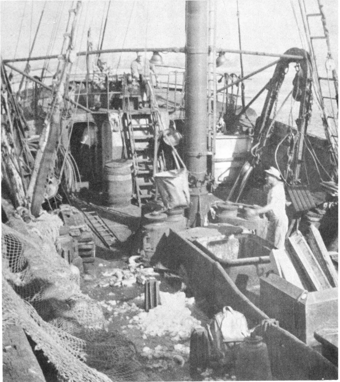
Figure 10.—Unloading fish from a hold of the ship by the use of a canvas basket and a winch. Note the basket in the air being swung out of the hold. (Boston, Massachusetts)
